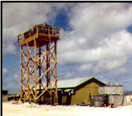
Water Tower & Power Shed
